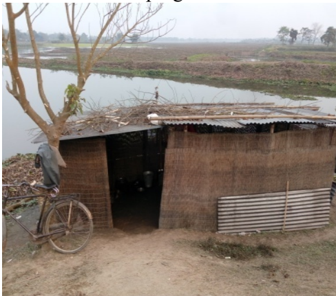
Fig.20: Baha , a Hut Constructed Near Beel
