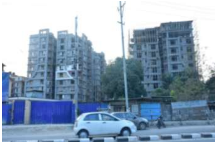
Under construction Apartment
