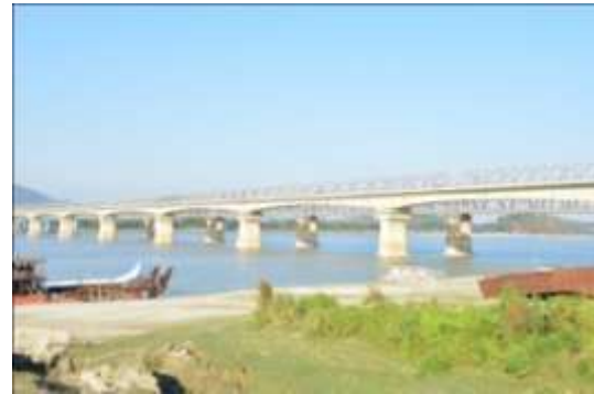
Brahmaputra River Bridge
