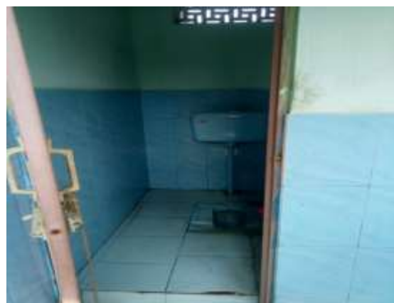
Toilet nad urinal facility
