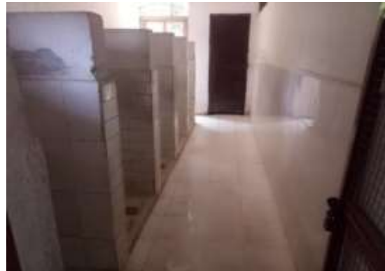
Toilet and urinal
