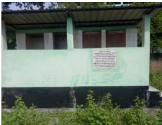
Toilet and urinal facility
