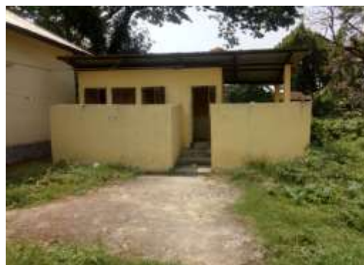
Toilet and Urinal
