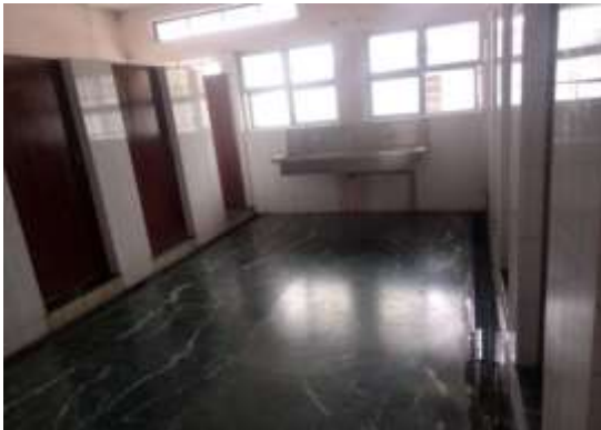
Toilet and Urinal facility
