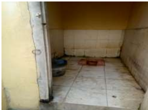
Toilet and urinal
